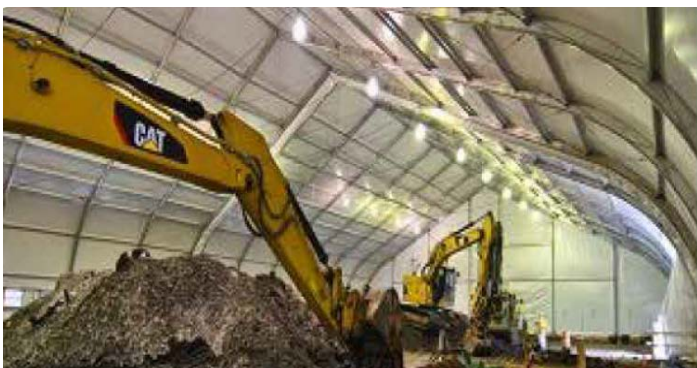
Soil Solidification inside tent (image courtesy of Honeywell)
