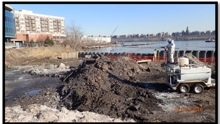
Worker applying Posi-shell.
